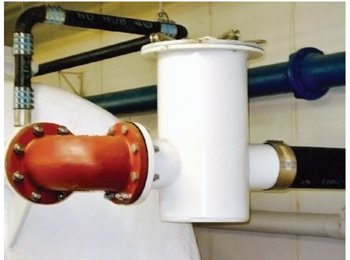
Dimensions for underground and aboveground cylindrical carbon steel sample port: 24" diameter x 16" height
