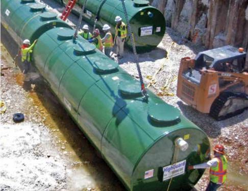
Highland Tank proudly manufactures the most extensive line of grease interceptors in the industry. We offer **automatic**, **gravity**, **flush-with-floor**, **and manual** grease interceptors to trap grease and solids before they enter a wastewater disposal system to help prevent sanitary system overflows. Municipal plumbing codes vary, so **we work closely with our partners** to offer customizable options where necessary.
