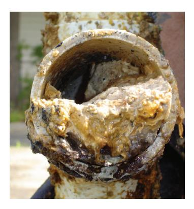
Designed to trap and collect large quantities of sewer-cloggir fats, oils, grease, and solids
