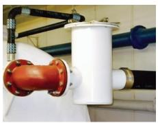
Efficient maintenance and operation of many wastewater treatment systems require sampling outflow for FOG concentration. Highland Tank offers interceptor-mounted, in-line and free-standing sampling ports to enable pretreatment inspectors to collect representative sample of the wastewater being discharged to the sanitary system.
