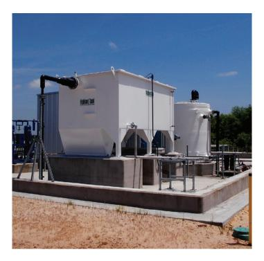
Rectangular oil/water separators can be installed aboveground to help industrial facilities comply with the EPA's spill and discharge regulations. Like our cylindrical underground units, these separators are equipped with our non-clogging Corella<sup>®</sup> coalescers that accelerate the separation process and greatly reduce the level of oil and oily-coated solids discharged into municipal storm or sanitary sewer.
