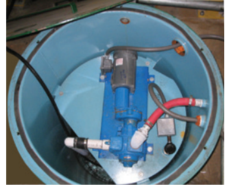
High-performance oil/water separator with influent pump packages
