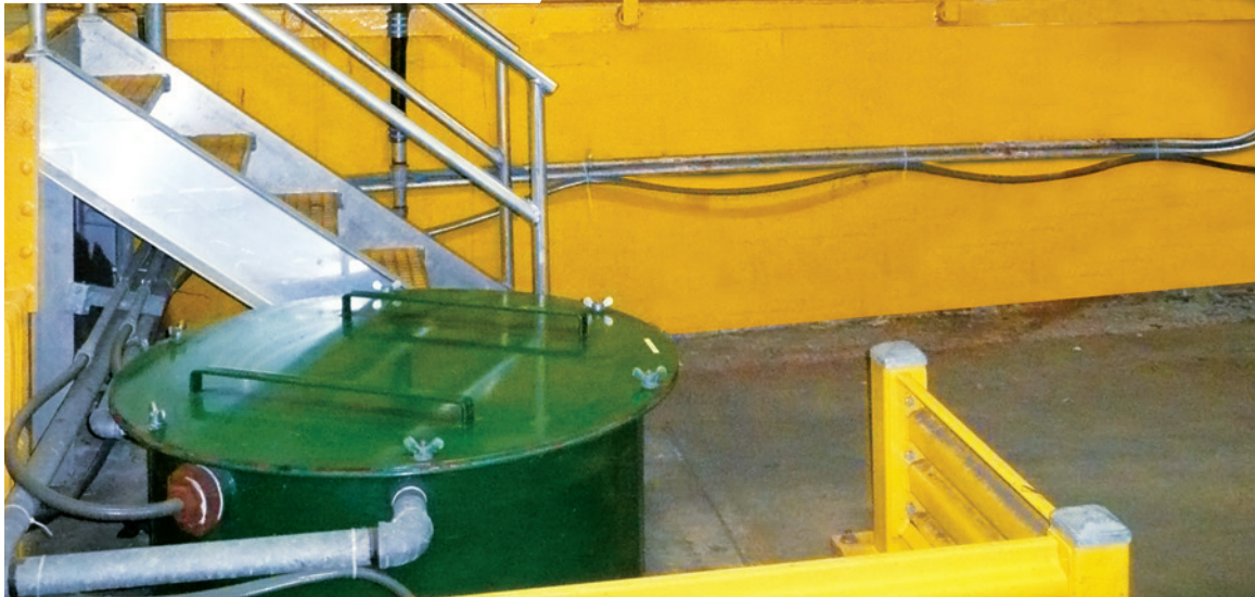
deep sump basin
