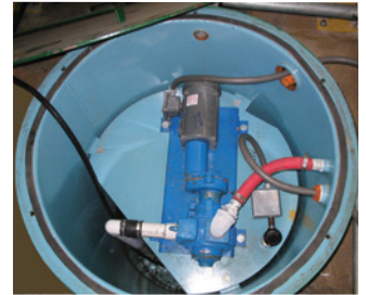
High-performance oil/water separator with influent pump packages
