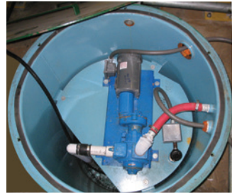
High-performance oil/water separator with influent pump packages
