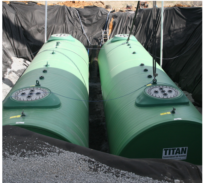
Two 20,000 gallon Titan® tanks with Sump Collars at a High's Store near Frederick.
