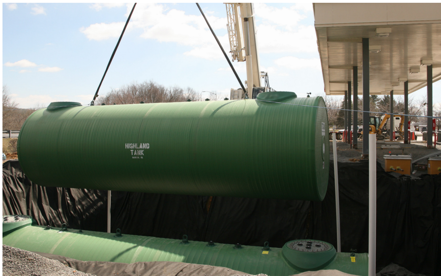
The second of two 20,000 gallon Titan® tanks lowered into excavation at a High's Store near Frederick.
