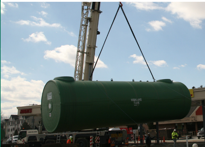
The Titan® is compatible with all motor fuels along with their ethanol, methanol, and MTBE additives.
