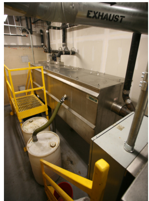
Automatic Grease Interceptor Units in use (right) and being constructed in our factory (bottom).
