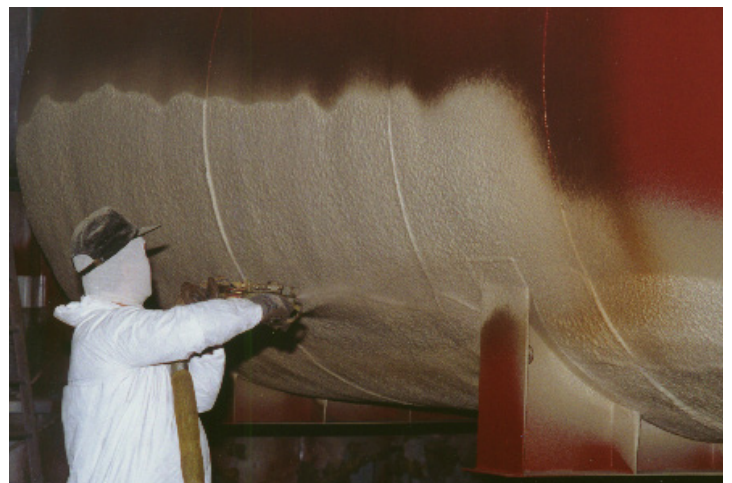
Injected or spray-on insulation system
