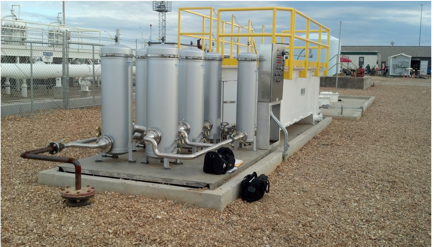
Advanced Hydrocarbon Filtration Systems (AHFS) are used in applications where hydrocarbon removal beyond the capability of a standard oil/water separator is necessary.
