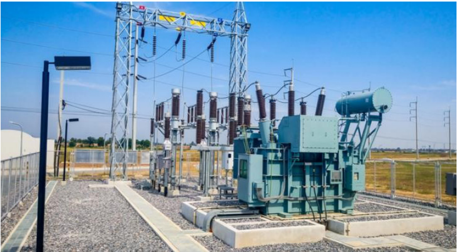
Oil-filled, substation transformers are used in electric power substations and in a wide variety of commercial and industrial applications
