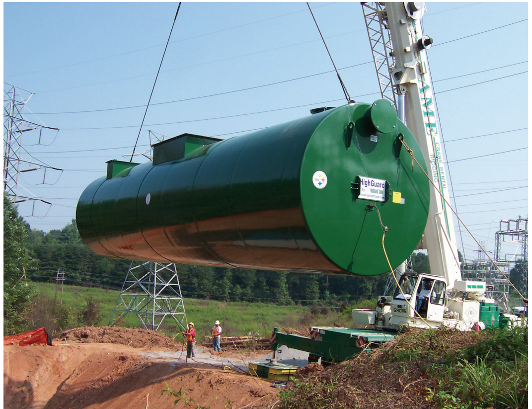
The Corella® oil/water separator is a stationary wastewater treatment tank, filled with water. It contains specially designed internal baffles and coalescers to accelerate the separation process.
