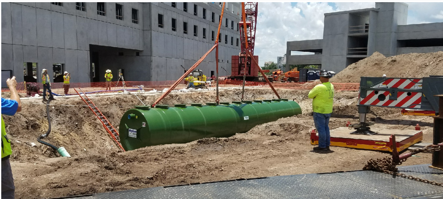
Highland Tank's gravity flow, multi-chamber passive grease interceptor.
