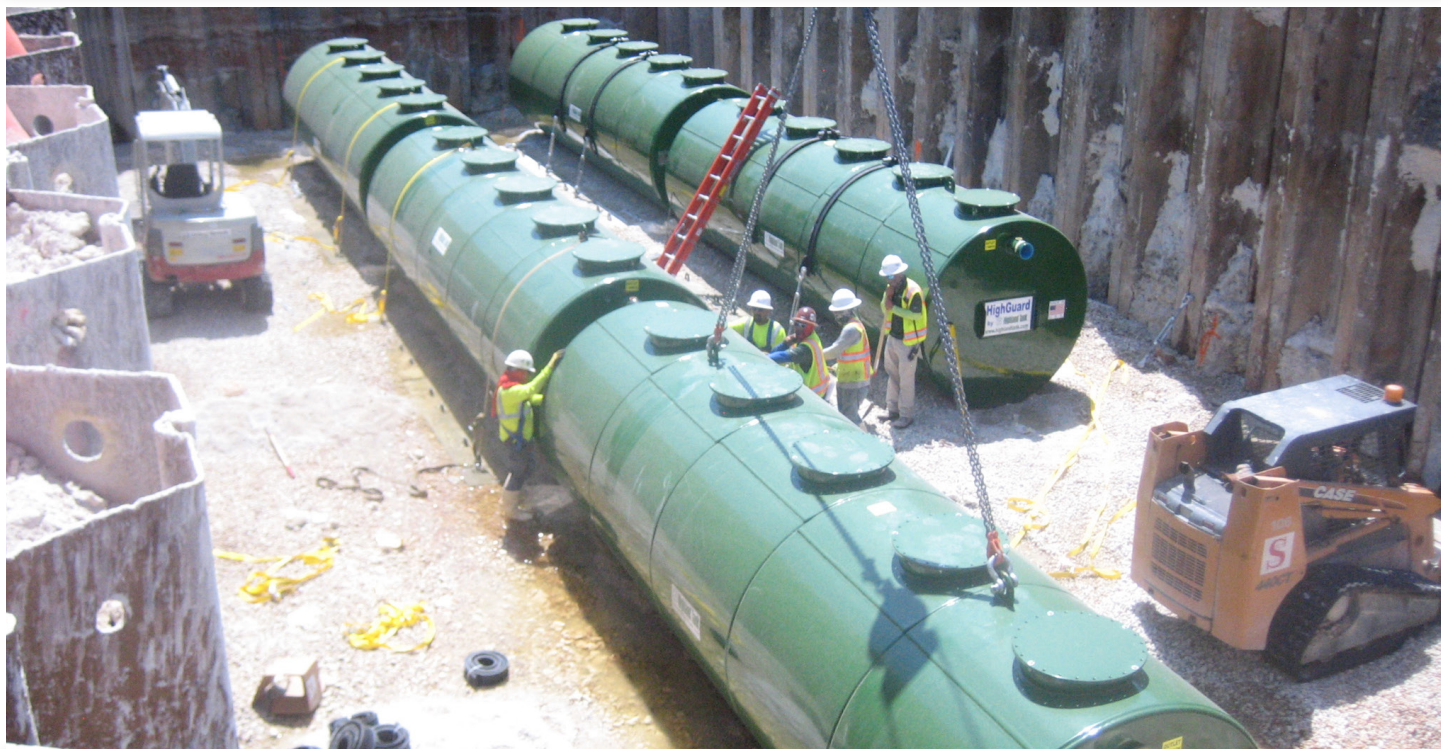
Highland Tank underground passive grease interceptors (PGI series).
