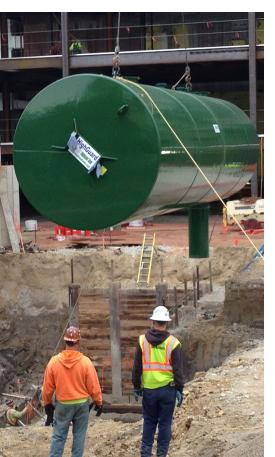
**Head Design:** Flat, flanged - standard Flanged and dished, or coned (vertical only) are also available
