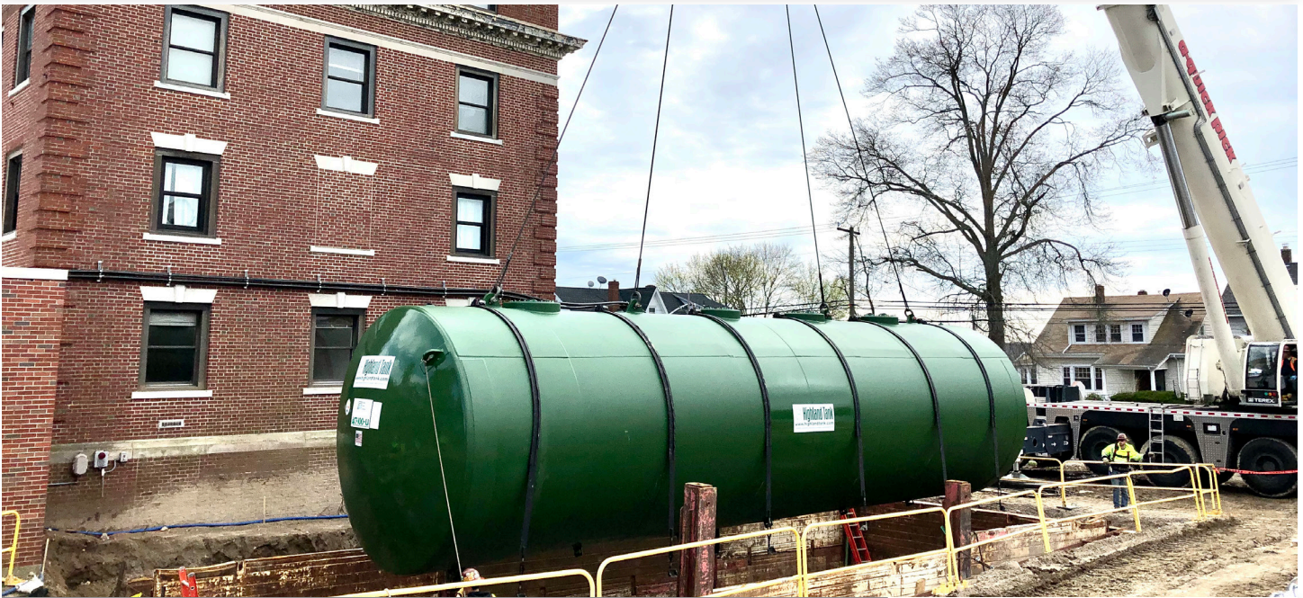
A 40,000 gallon fuel storage tank is being installed at a hospital.
