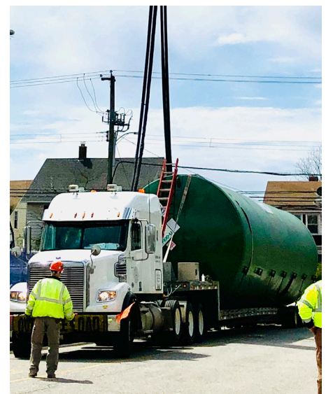
A Highland Tank truck delivers the 40,000 gallon fuel storage tank.
