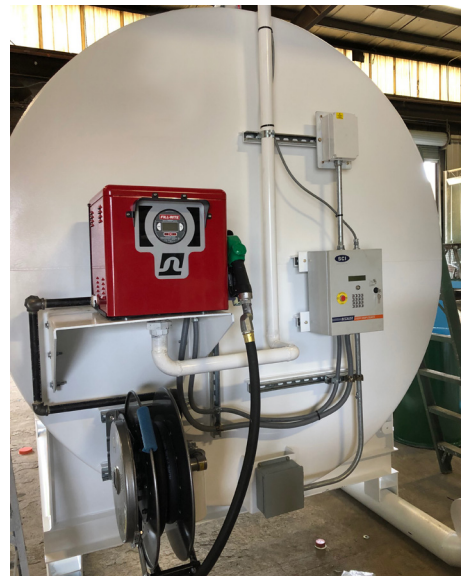
The photo above shows a Tier II system with pump and meter mounted on tank head.
