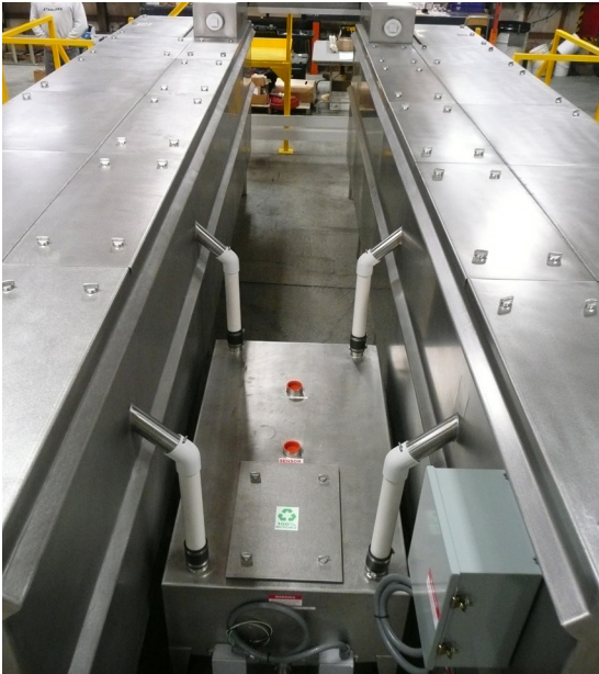
The photos above show two large volume automatic grease interceptors (left), a small, under-sink automatic grease interceptor in a kitchen (top center), a single-basin passive grease interceptor (bottom center), and a triple-basin passive grease interceptor.
