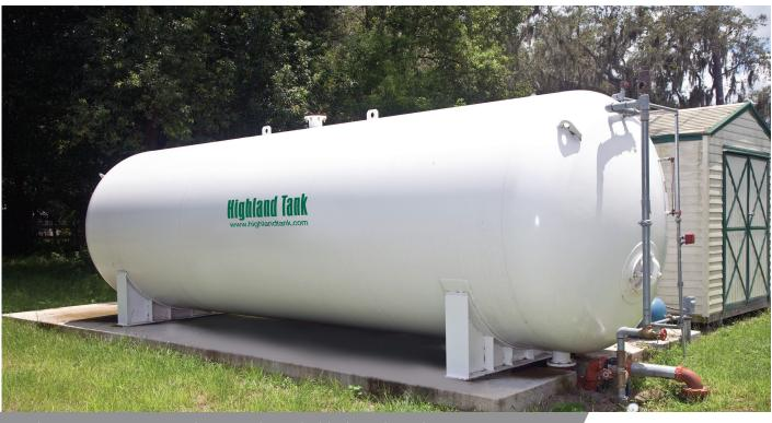
Chlorine Contact Tanks (CCT) are typically used with chlorine injection equipment in a well water system to help comply with strict new drinking water standards
