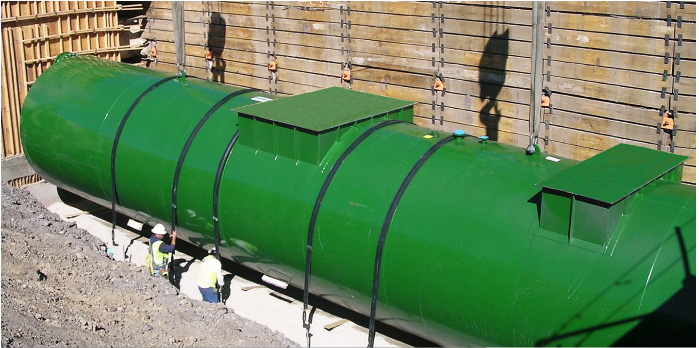
Oil/water separators for spill control and discharge compliance shall be provided in conjunction with the trench drainage systems serving all aircraft storage and servicing areas.
