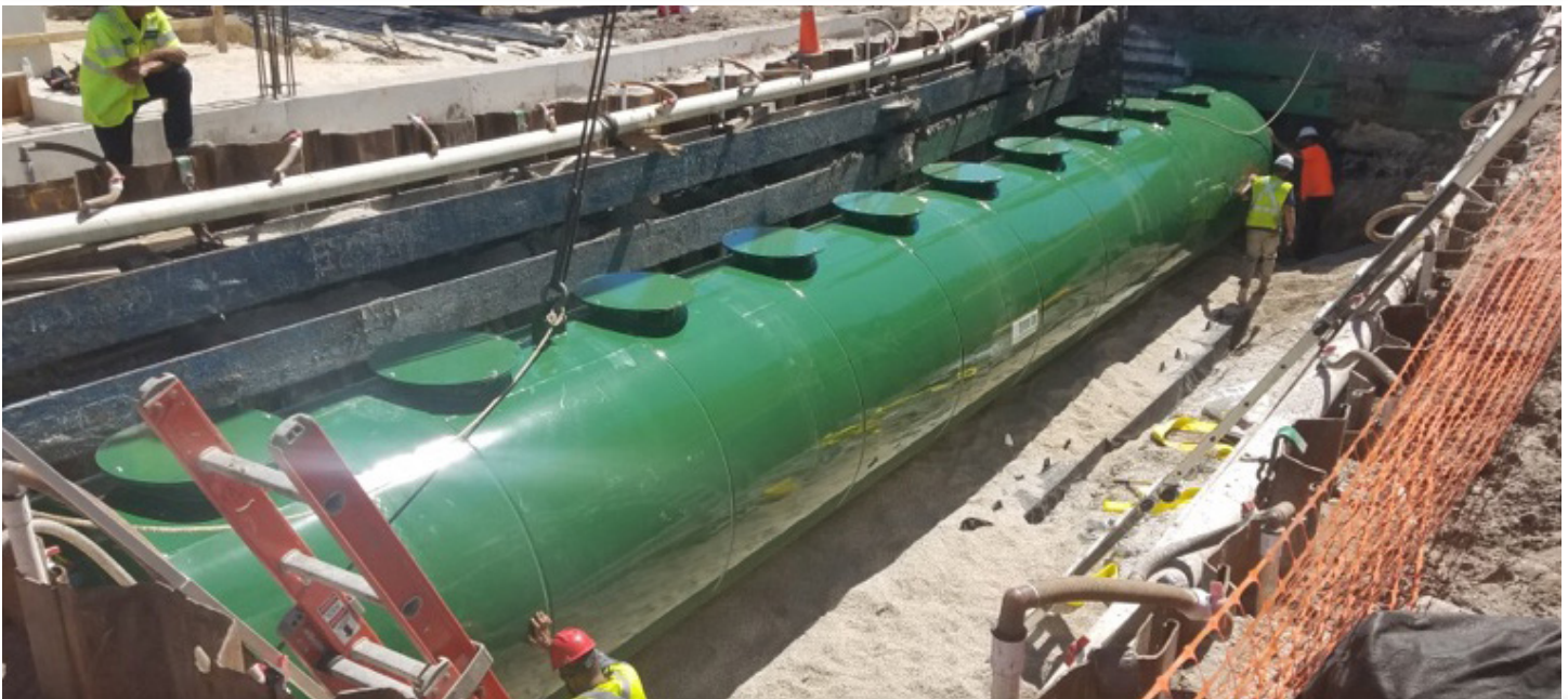
Highland Tank's multi-chamber, gravity-flow passive grease interceptor.
