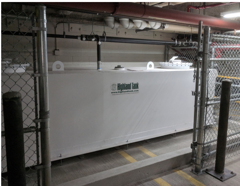
Highland Tank's Passive Grease Interceptors can be installed in parking garages for easy pump-outs.
