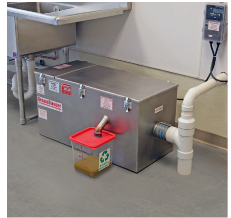
Highland Tank's point-of-use GreaseStopper® Automatic Grease Interceptor can fit under wash sinks.
