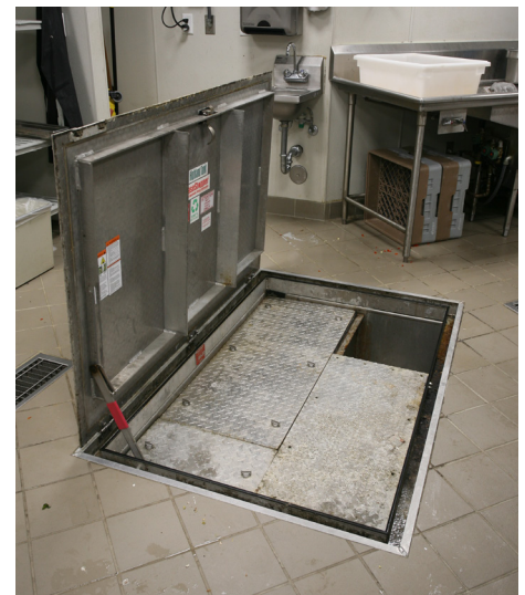
Highland Tank's flush-in-floor GreaseStopper® AGI installed in a kitchen floor with a non-skid stainless steel access door.
