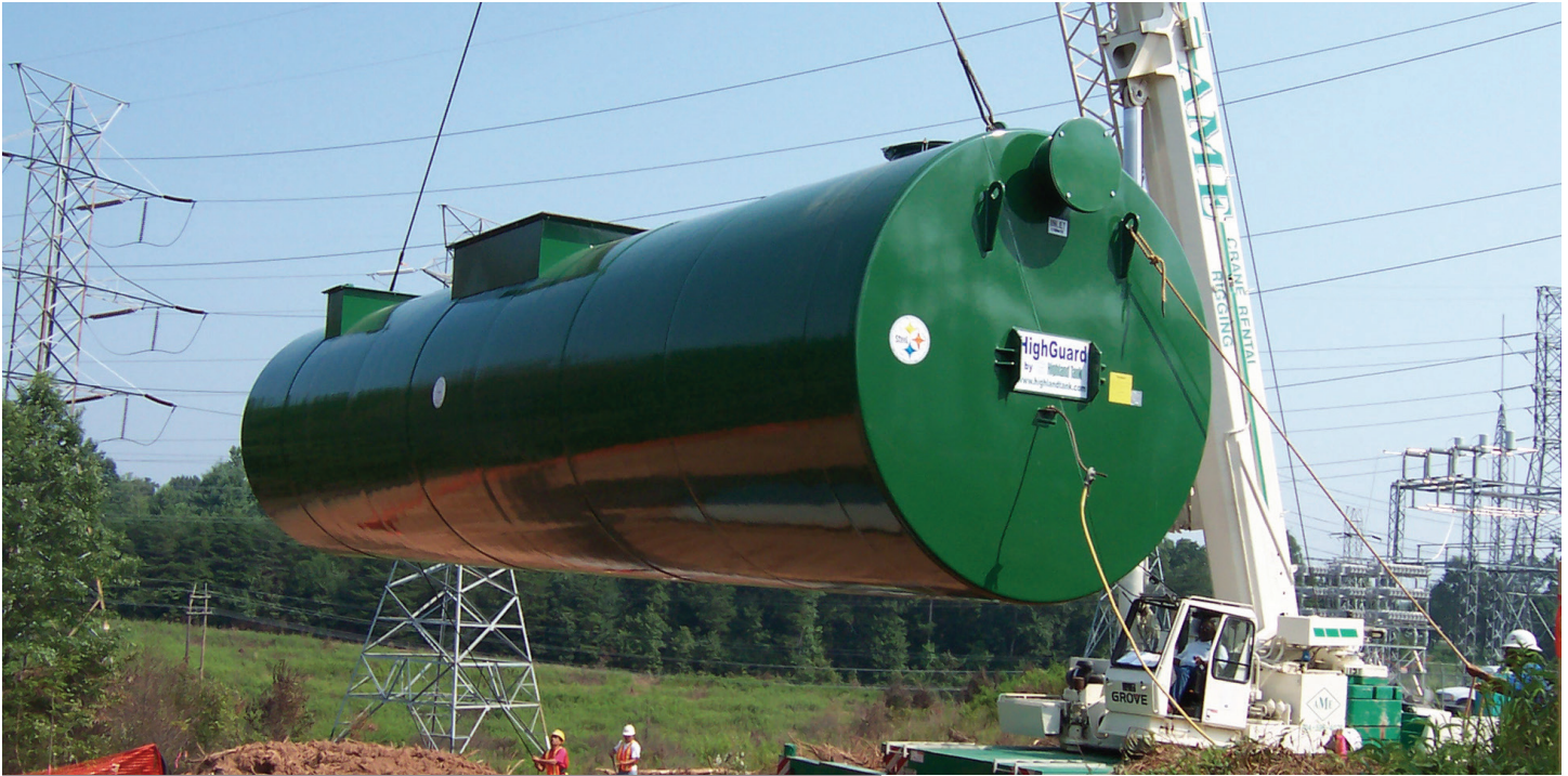
A Highland Tank 40,000 gallon oil/water separator is installed at a power facility.
