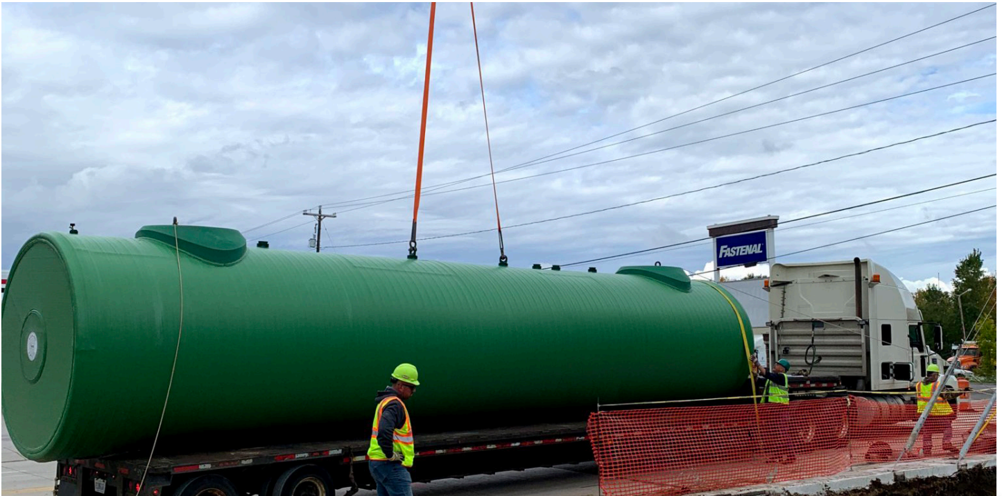
Titan Tank installation at a new convenience store.
