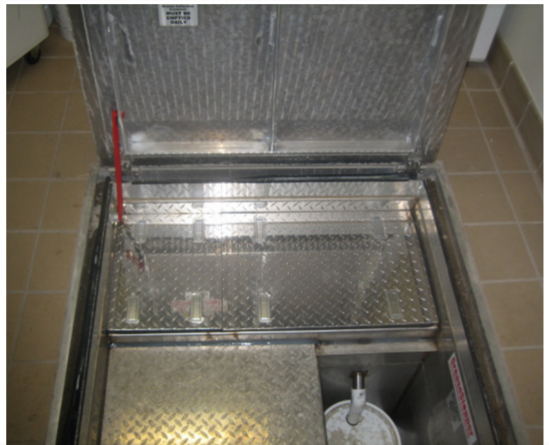
The flush-with floor automatic grease interceptor (shown on right) eliminates the need for costly service as well as odors.
