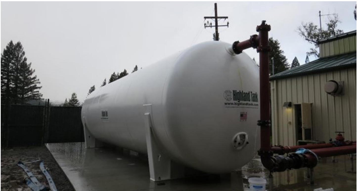
Chlorine Contact Tank System for EPA 4 Log disinfection
