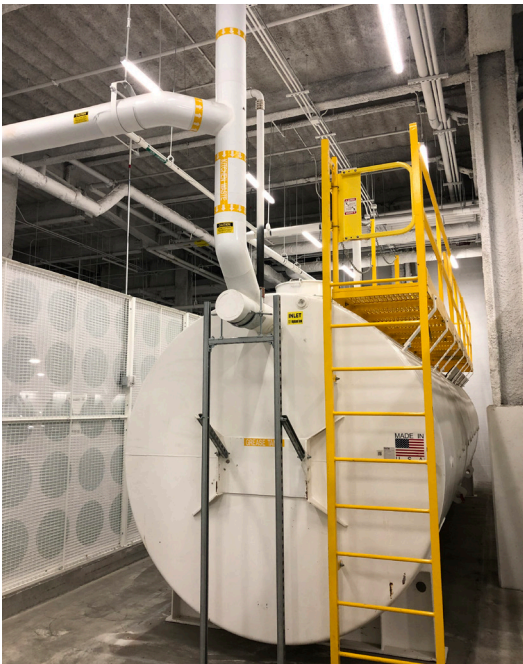
Passive Grease Interceptors (PGI) installed in Boston
