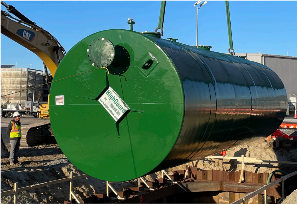
The HTC-G-20,000 gallon OWS is lowered into the pit at the installation site.
