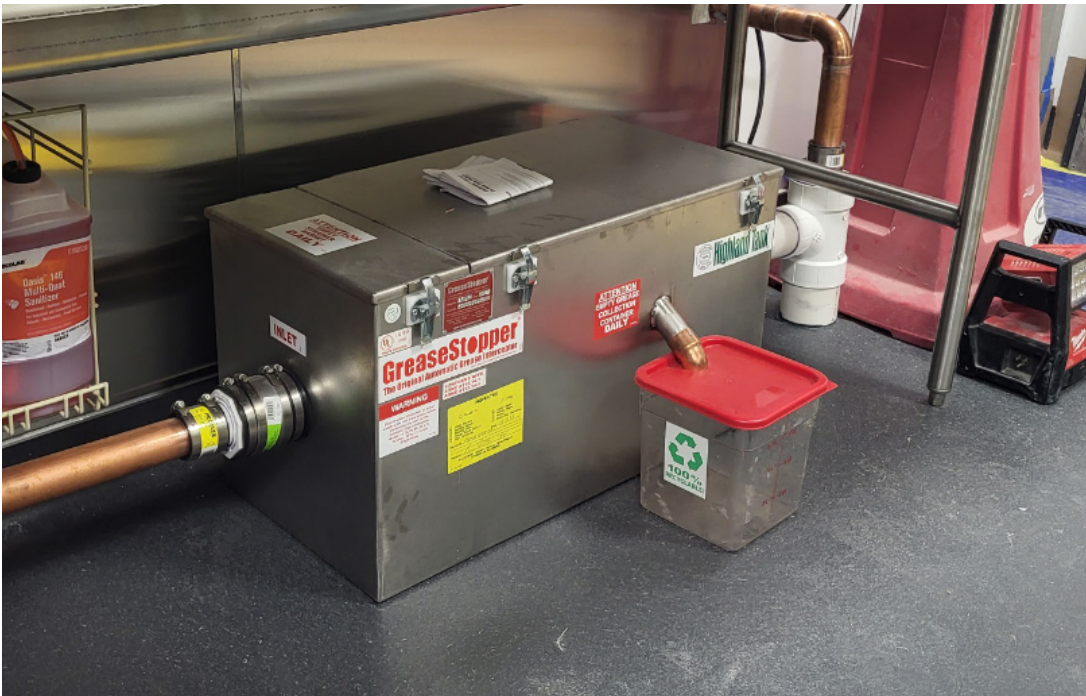
Highland Tank automatic grease interceptors reduce costly maintenance fees.
