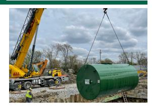
The HighGuard underground storage tank features two steel walls with a strong dielectric coating of high solids polyurethane for protection, even under the most difficult conditions. HighGuard resists surface damage due to impact or abrasion that may occur during transportation, rigging and installation.
