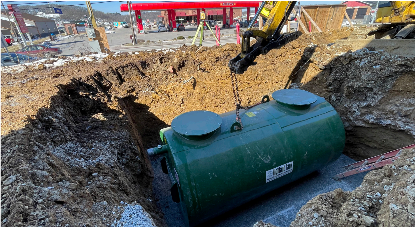
Highland Tank manufactured two 1,500 gallon double-basin PGIs for a food plaza opening in Pennsylvania.
