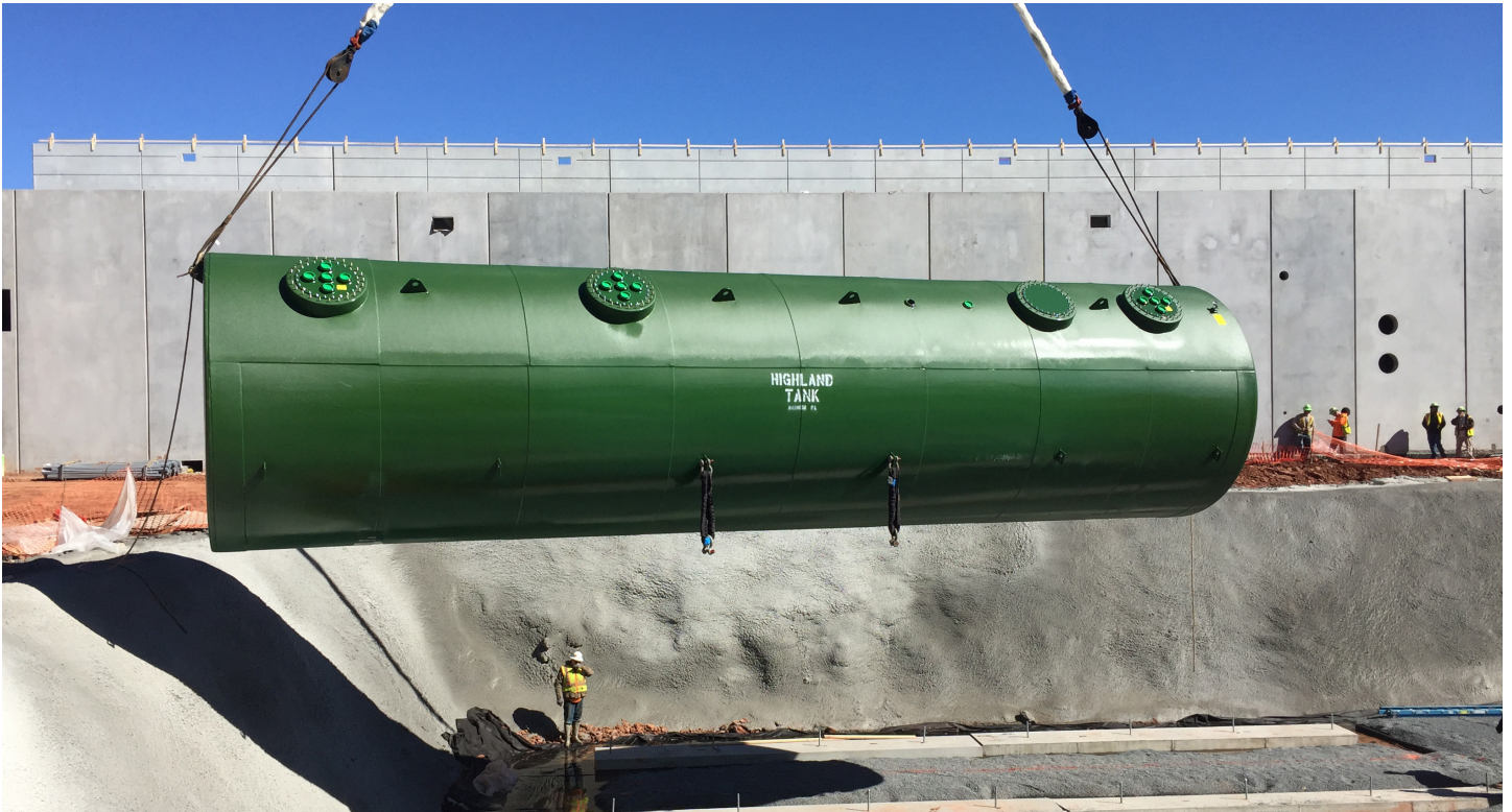
Highland Tank HighGuard protected underground steel storage tanks for a data center.
