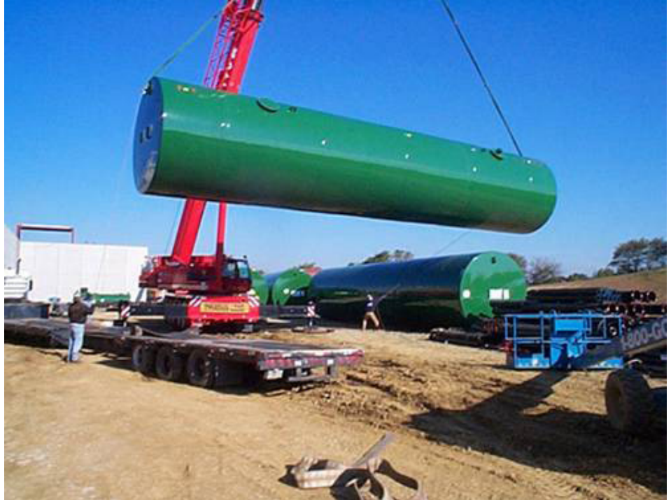
Highland Tank HighGuard protected underground steel storage tanks for fuel storage.
