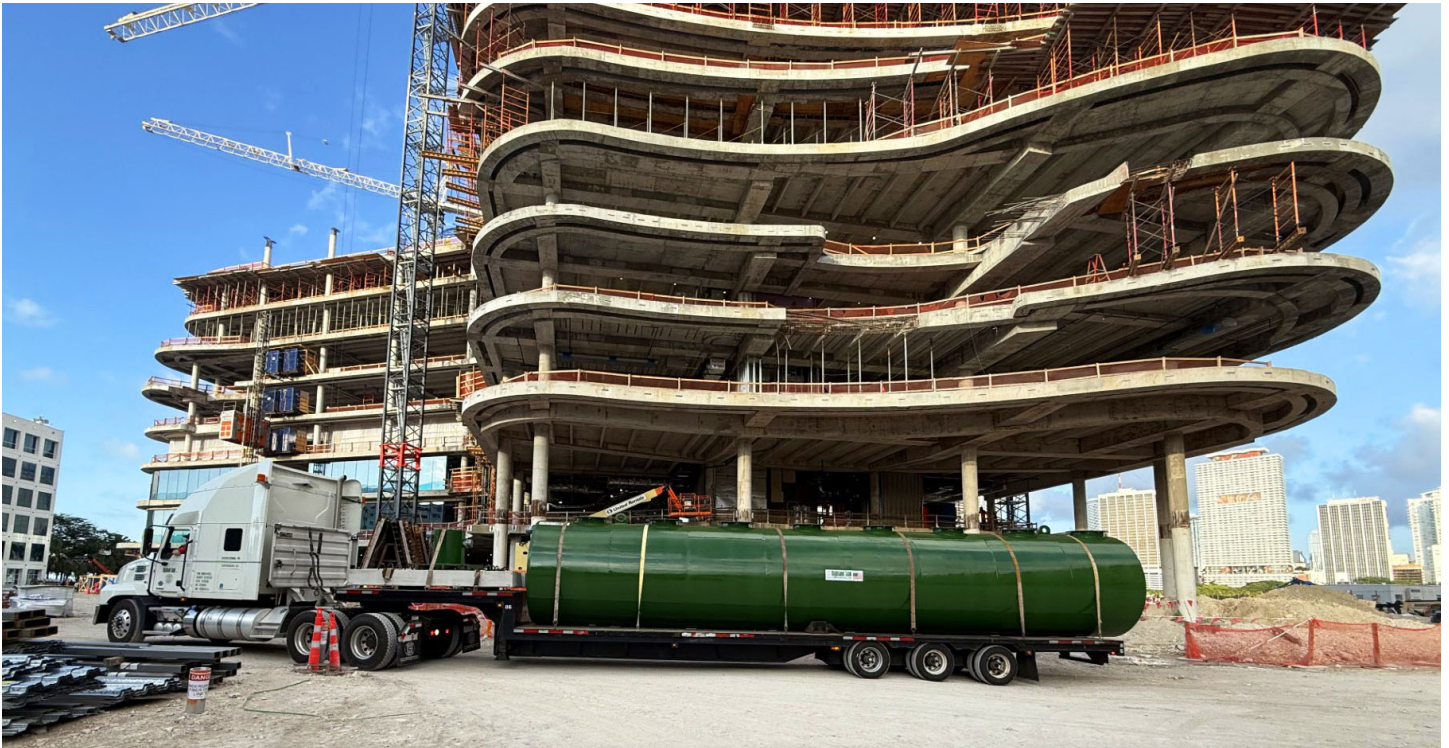
10,000 gallon Passive Grease Interceptor with 8 chambers
