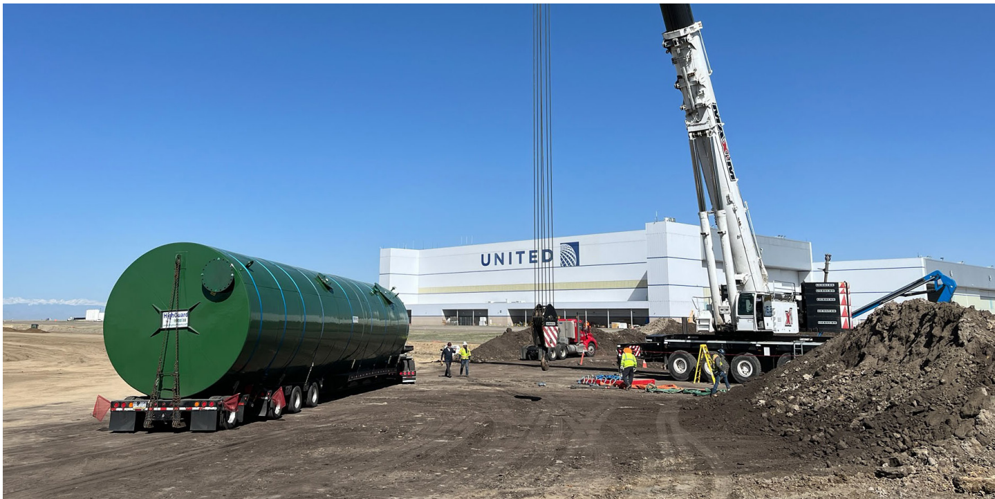
A 50,000 gallon Oil/Water Separator arriving for installation at airport
