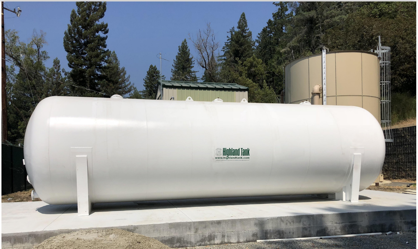
Chlorine Contact Tanks (CCT) are typically used with chlorine injection equipment in a well water system to help comply with strict new drinking water standards.
