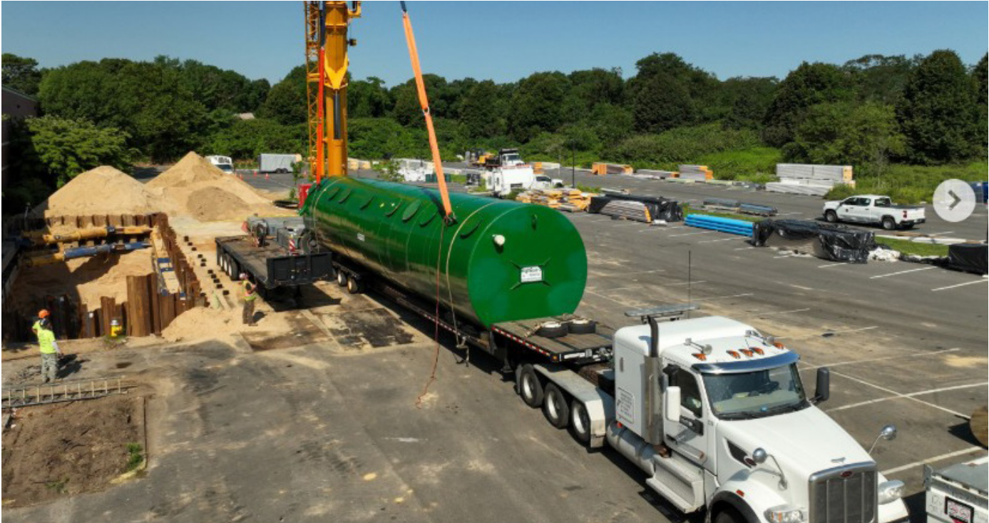
This 50,000 gallon passive grease interceptor was installed at a food manufacturer and distributor.
