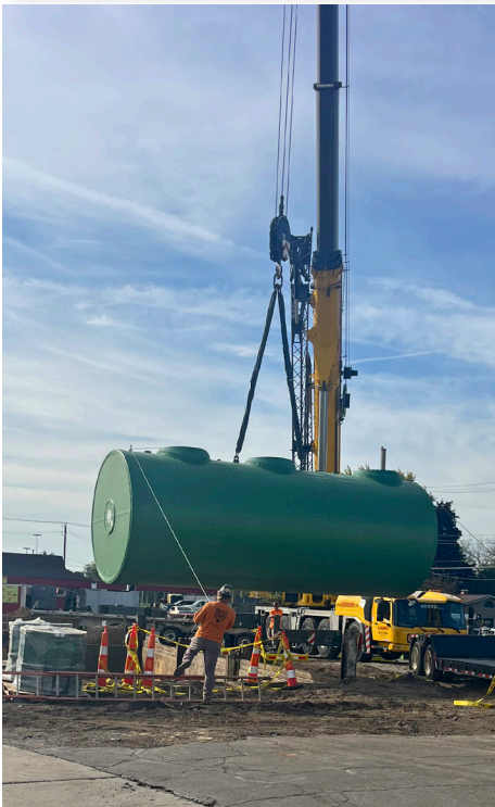
The above photos show a 15,000 gallon TITAN® tank split into three 5,000 gallon compartments.
