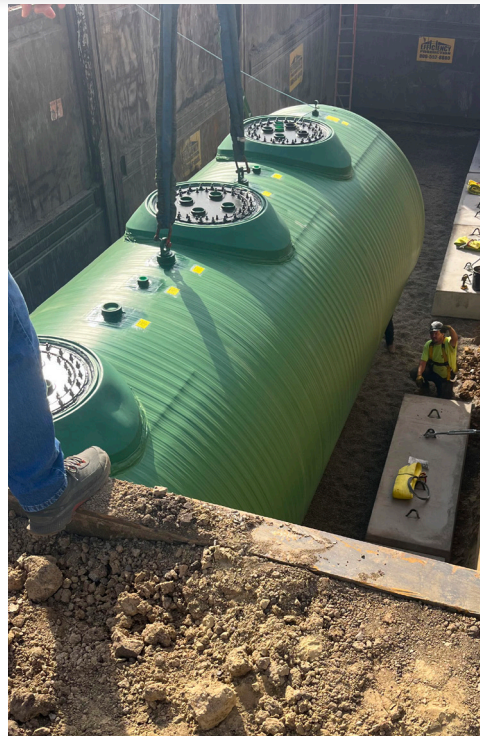
The above photos show a 15,000 gallon TITAN® tank split into three 5,000 gallon compartments.
